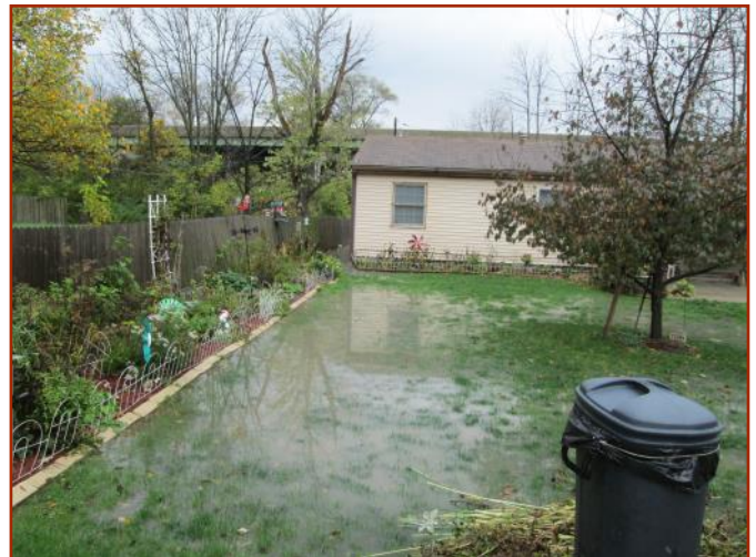
Poorly drained soil types and poor surface drainage can lead to drainage & flooding problems during wet months of the year.
