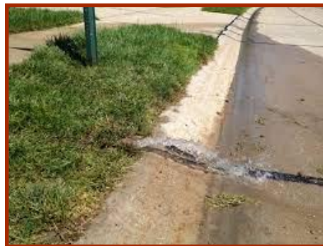
Discharging sump pumps to the curb is illegal & creates a safety hazard.
