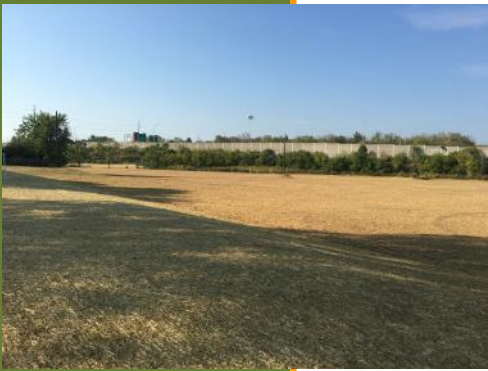
This site, properly mulched & dormant seeded is ready for winter.
