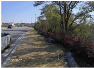
Construction Site Reviews and Inspections Help Prevent Pollution
