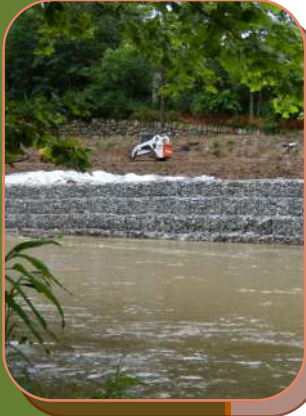
Gabion Baskets are one form of erosion control for extremely critical areas of a stream
