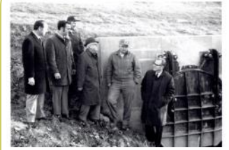
1971 - District Conservationist Ken Pyle & Supervisor Leroy Murphy assist with major flooding problem solution.
